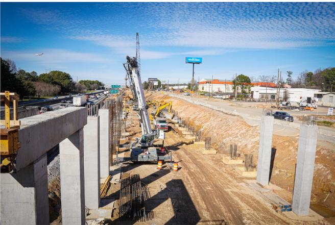
"The project is approximately a mile of connected C-D lanes, connected distributor lanes, I-75 C-D lanes and I-75 connected distributor lanes," said Pablo Giraldo, a Walsh Group project engineer. "We're pretty much widening I-75 in an existent frontage road to the outside to create better flow for the interchange that is at the end of the project."
